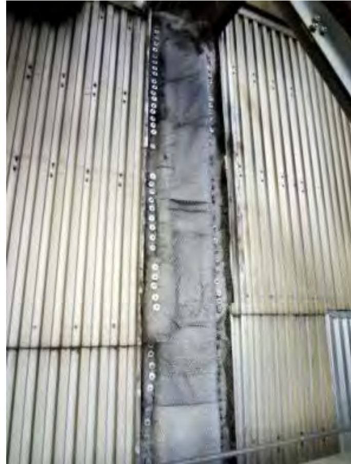
Original ISOMEMBRANE® Installation in 1996, photos taken Jan 2013
